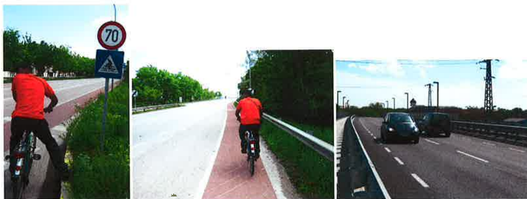
Figure 4: Other observations made during the site visit
