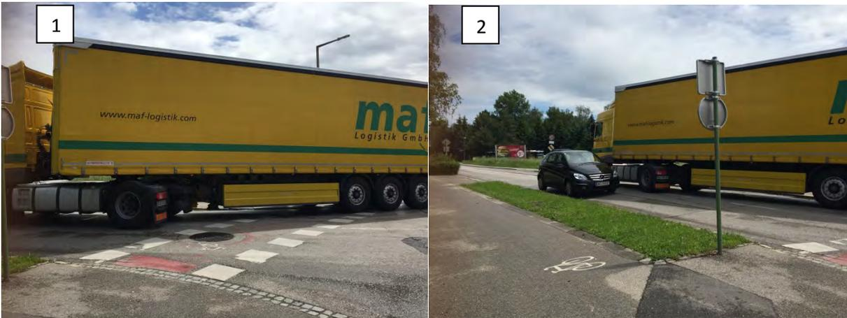
Figure 2 show short turning lane , the big truck will be blocked when turning
