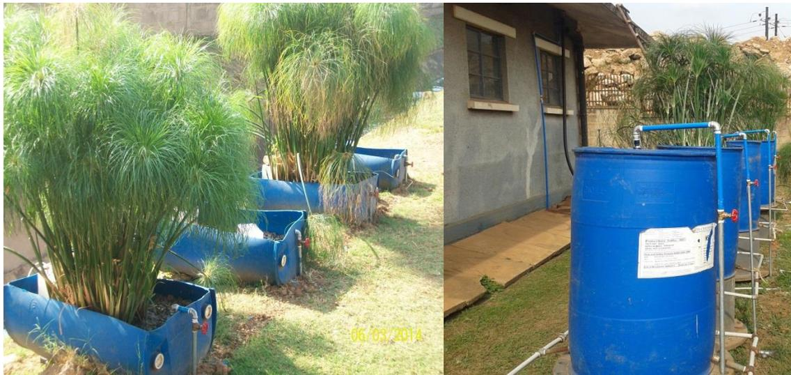
Figure 4: Horizontal (left) and Vertical (right) subsurface flow constructed wetland mesocosms designed as buffer strips for organic matter and nutrient removal from municipal WWTP effluents. Source: Field photos by Najib Bateganya
