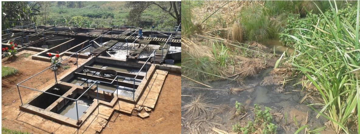
Figure 3: Dilapidated Masaka WWTP (left) and WWTP effluent-wetland stream confluence (right). The WWTP effluent is characterised by the black colour at the effluent-wetland stream confluence. Source: Field photos by *Najib Bateganya*
