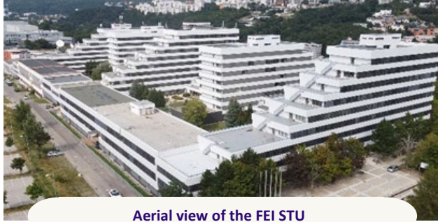
Aerial view of the FEI STU
