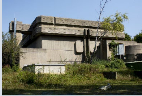
North wing before renovation
