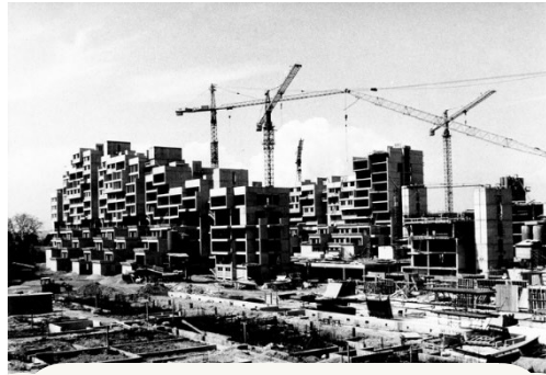
During the construction
