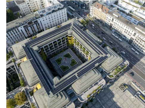
Fig. 9: PV – systems on the roof; https://www.linz.at/stadtentwicklung/128011.php
