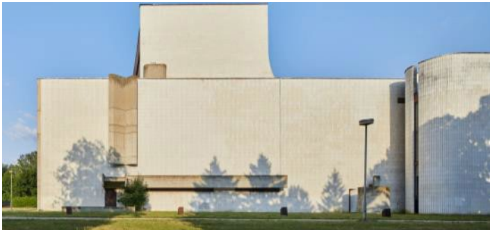
Side of the building
