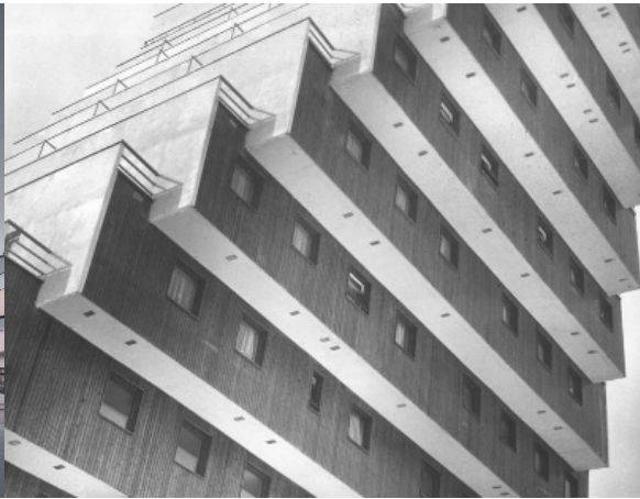
Close up of the floor composition before renovation
