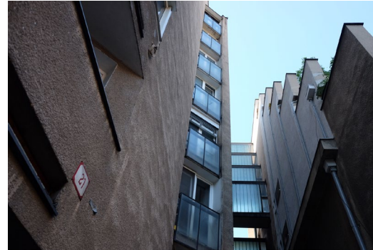
Fig. 3: Backside of the building
