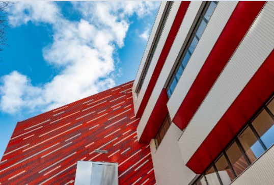
Red aluminium slats on the extension
