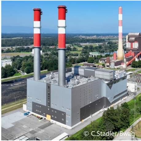
Gas power station Mellach (838 MW)
