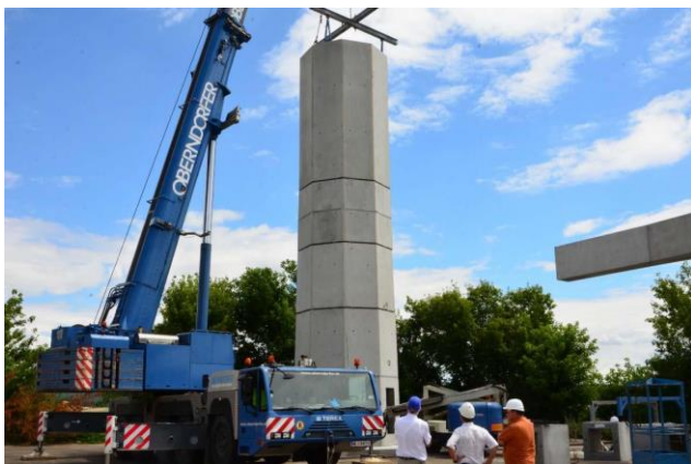
Prototype erected using the new construction method
