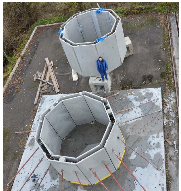
Two double-wall construction segments
