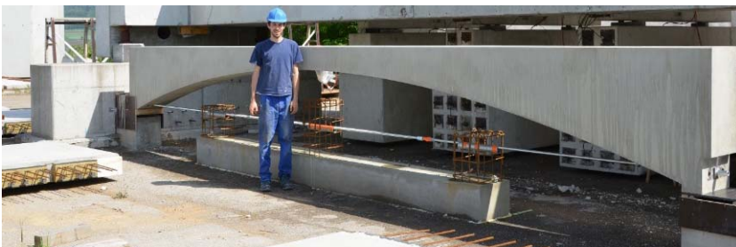
▼ Construction of a prototype to test the new technology
