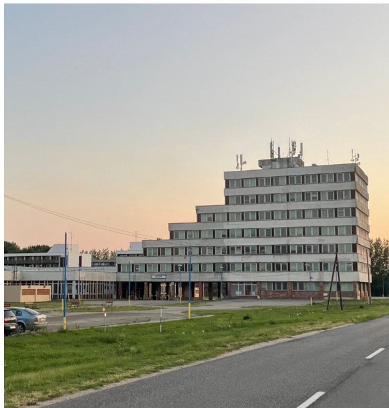
Accommodation building in Gabčíkovo. / STU
