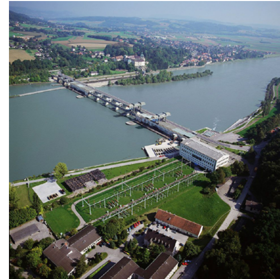
Ybbs-Persenbeug hydroelectric power station. Austria / VERBUND, UWK
